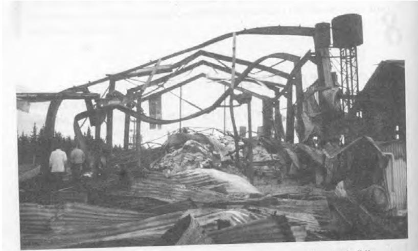
**Figure 2.26 Steel Structural Failure due to Fire**
