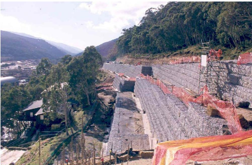
Figure 3 illustrates a landslide with a large footprint but with a low angle failure. The trigger for the landslide was high water content of the material forming the slope. Elements of the landslide have been recorded as becoming mobile during periods of extended wet weather during the last 10 to 15 years.
